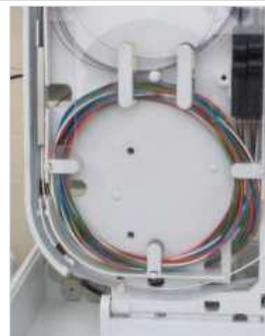
Lead output pigtail to other side of the tray, then insert adapter as picture displays.
