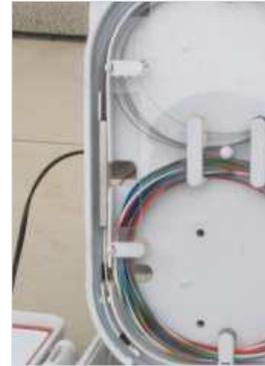
Splice splitter with output pigtailed.
