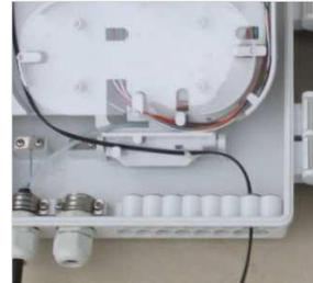
Pre-installed filed assembly connector of a drop cable, then insert connector to optical adapter in order and tie it with cable ties.
